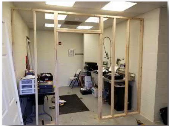
Constructed a new wall in Amp concessions
